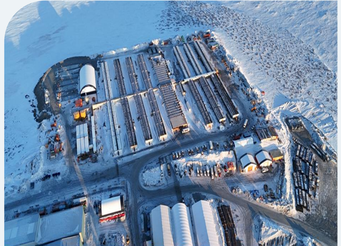
◆ Goose Project Accommodation Complex – April 2024
